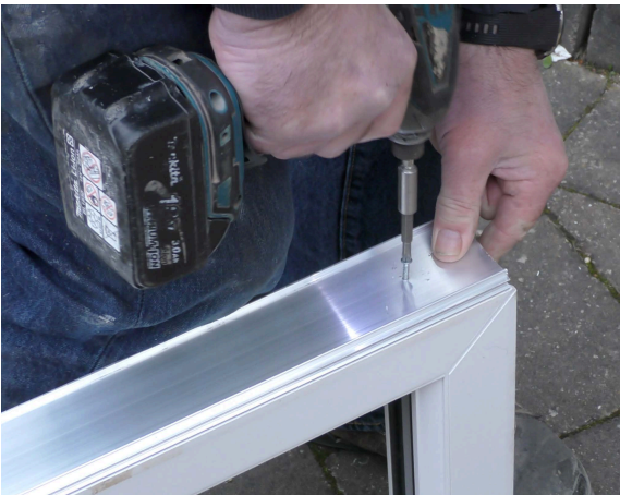
Measure, cut and fix the coupler to the light.
