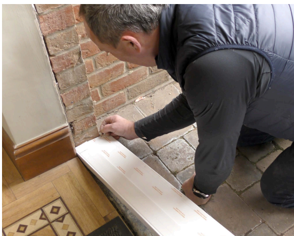
Measure and cut the cill to the required size, taking into account for cill horns if desired.
