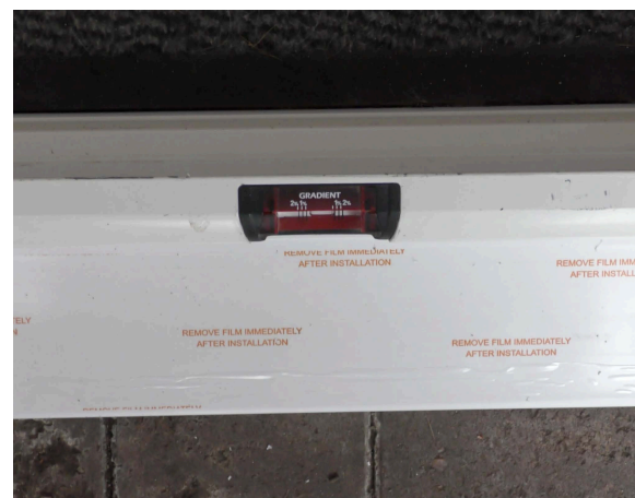
Ensuring the hinge side is slightly higher than the closing side, will give you a head start when toe and heeling the door.
