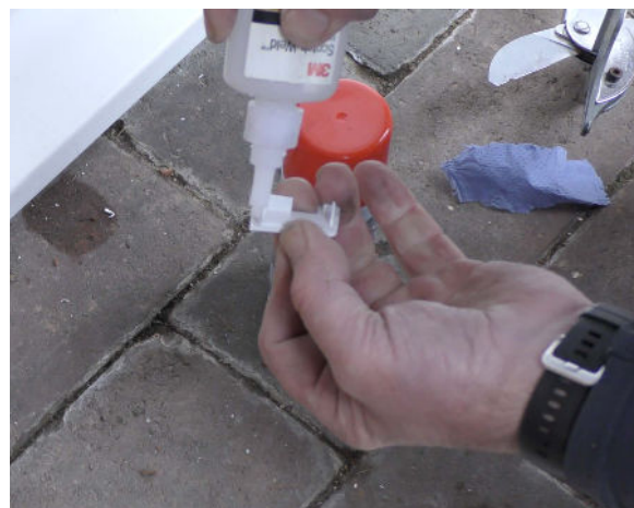
Attached the cill end caps using adhesive to seal and fix in place.
