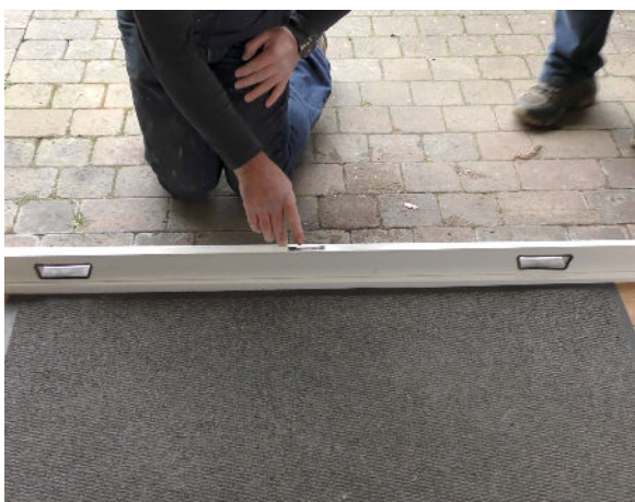
Place the cill on to the aperture. Use a spirit level to assess the level of the cill. If required, place packers under the cill, check the level and adjust if necessary.
