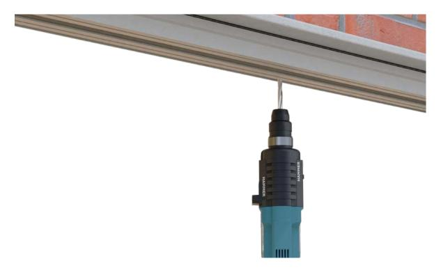
Drill and countersink an appropriate sized fixing hole through the frame. This should be no more than 200 mm from the external corner of the frame.
