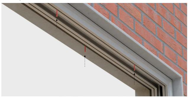
Where possible, fixing points should be on both sides of the frame, in a zig-zag pattern.
