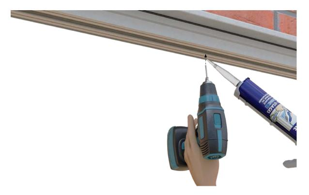
Insert suitable sealant to fixing hole, ensuring fixings are within 900 mm intervals, then screw preferred fixing in place.
