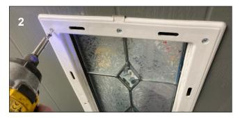
Remove the screws and inner mid piece. Ensure the glass is supported and does not drop out.
