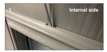
Insert a flat headed screwdriver into the prising slot and gently twist clockwise until the internal cassette starts to come away.
