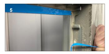
Place new gel tape around the retaining external cassette, remove the gel tape cover and gently position the glass against the external cassette.
