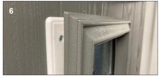
Fix the inner mid piece into position and insert all screws. Clip the outer cassette onto the inner mid piece.
