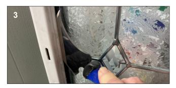
Use a moon knife to seperate the glass from the gel tape on BOTH internal and external sides. Remove all original gel tape and ensure the area is clean.
