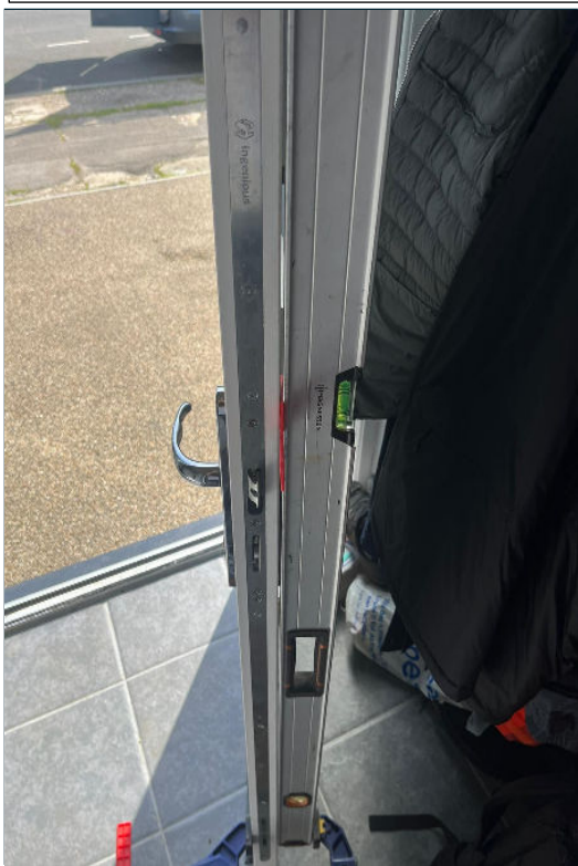
3. Close up of packer and straight edge.
